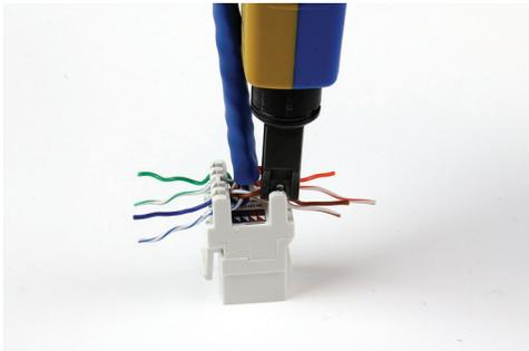
2. Place the wires into the keystone jack, setting the wire pairs into the IDC according to the displayed wiring configuration (A or B) and punch down the connections.
